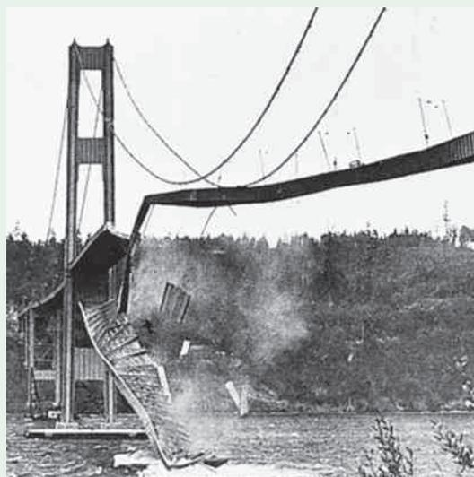
The Tacoma Narrows Bridge collapsed when winds set up resonant vibrations.
